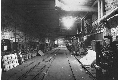
Tunnel - A One of the two parallel tunnels
